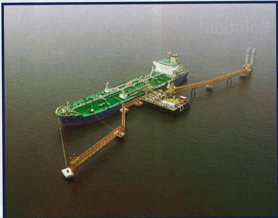
LPG berthing station 3-km offshore Peru, linked to the shore via ITP's subsea pipelines.
