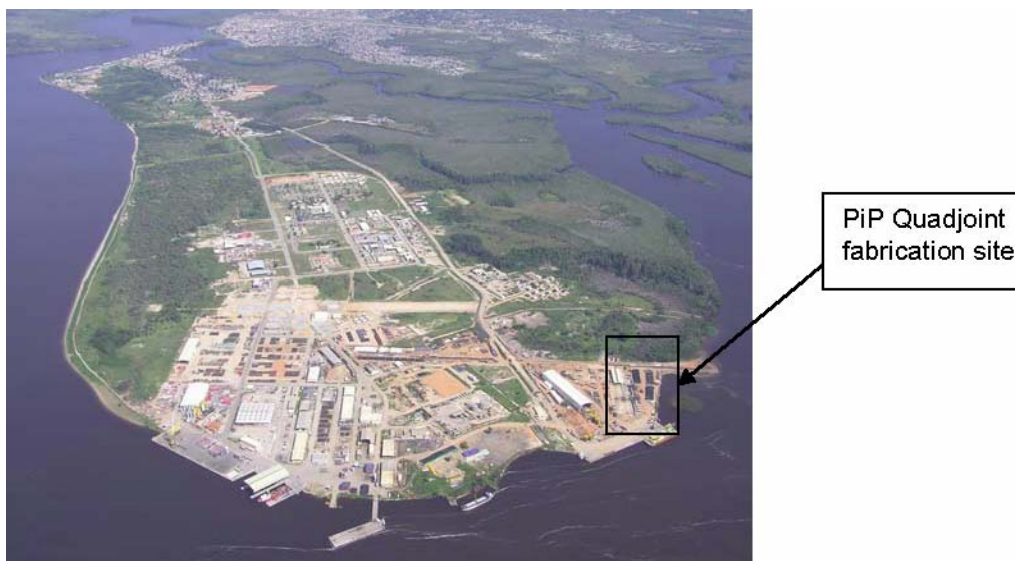
Figure 2: General view of Kwanda base. The three dark shapes are finished quad-joint
