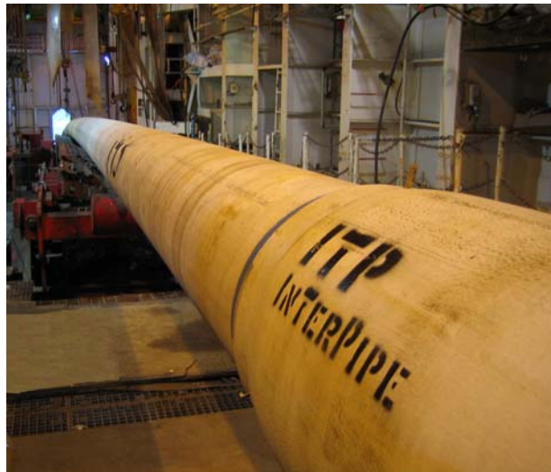
Fig 10: Pipe-in-Pipe field joint entering the overbend region
