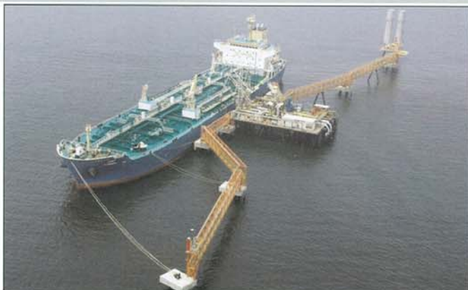
Figure 1 Camisea berth with subsea pipelines connecting to the onshore plant
