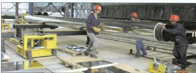
Figure 2 Onsite fabrication of pipe-in-pipe sections
