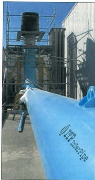
Figure 5 Full scale test section installed at SBM's facility in Nice, France
