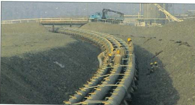
Figure 3 Flat pack containing pipelines and buoyancy modules during installation
